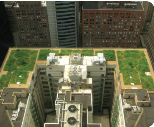
Vegetables, herbs, grasses, moss and decorative plants can all be grown on correctly prepared rooftops. A green roof provides excellent insulation and helps modulate the temperature inside the building. TONYTHETIGER/WIKIPEDIA.ORG
